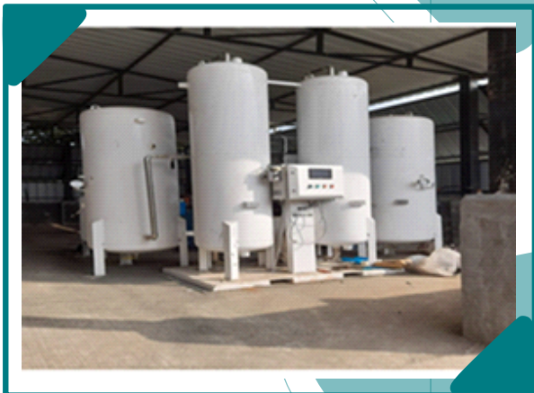
Oxygen Generation Plant
